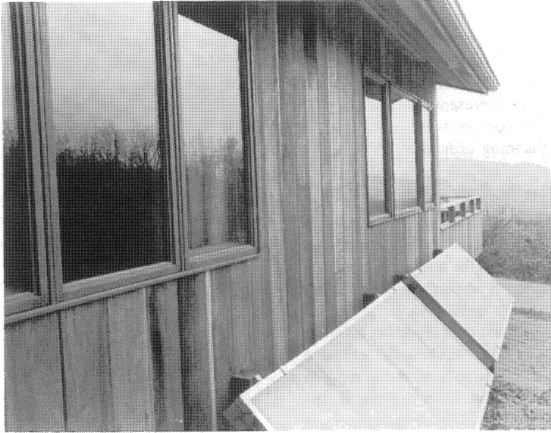
South windows of the master bedroom (left) and survival zone. Solar hot water panels provide summer shade for large glass areas of basement level.
